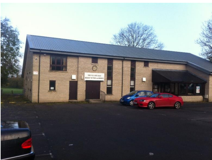
Picture 33 Village Hall on Wick Rd
