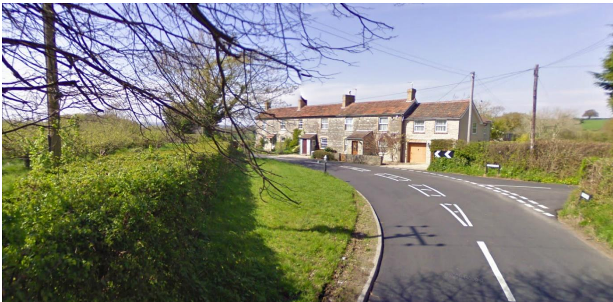
Picture 18 Older terraced cottages showing use of local stone & clay roman roof tiles
