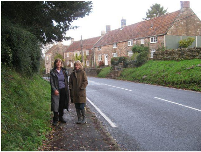
Picture 40 Stowey showing older terraced cottages, built in local stone, with clay roman roof tiles & survey team
