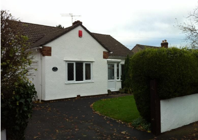
Picture 9 Rendered finish, roman roof tiles
