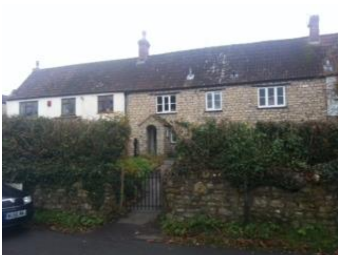
Picture 24 Terraced properties Stitching Shord Ln, set back & screened from road by planting
